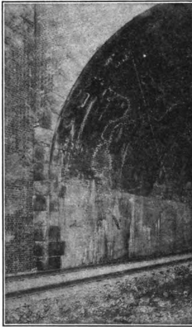
A SECTION OF TUNNEL CONSTRUCTION.
